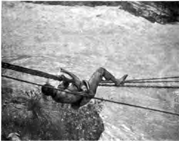
NATIVE CROSSING ROPE BRIDGE
